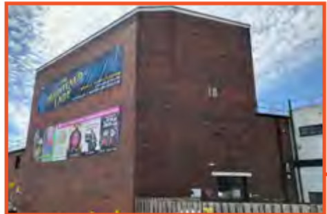
The fly tower of the theatre creates a challenging site edge
