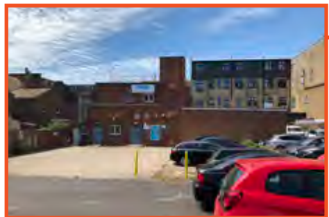
Parking areas of adjoining properties possess access rights on the site
