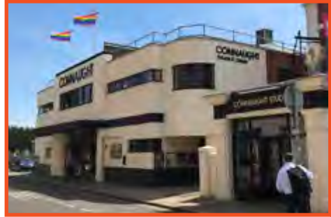
The art-deco style Connaught Theatre provides a strong anchor point for the site
