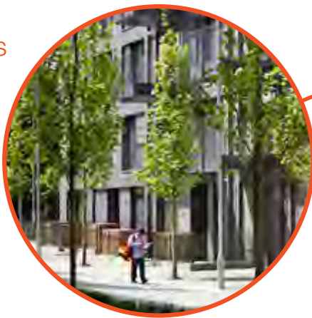
Active residential frontage St John's Hill, Wandsworth Hawkins\Brown
